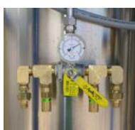
Dual Relief Valve Assembly
